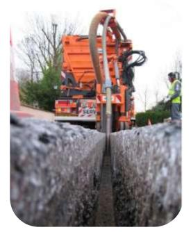
The Cleanfast machine cuts a narrow microtrench, simultaneously removing all spoil by suction to its integral storage bucket.
